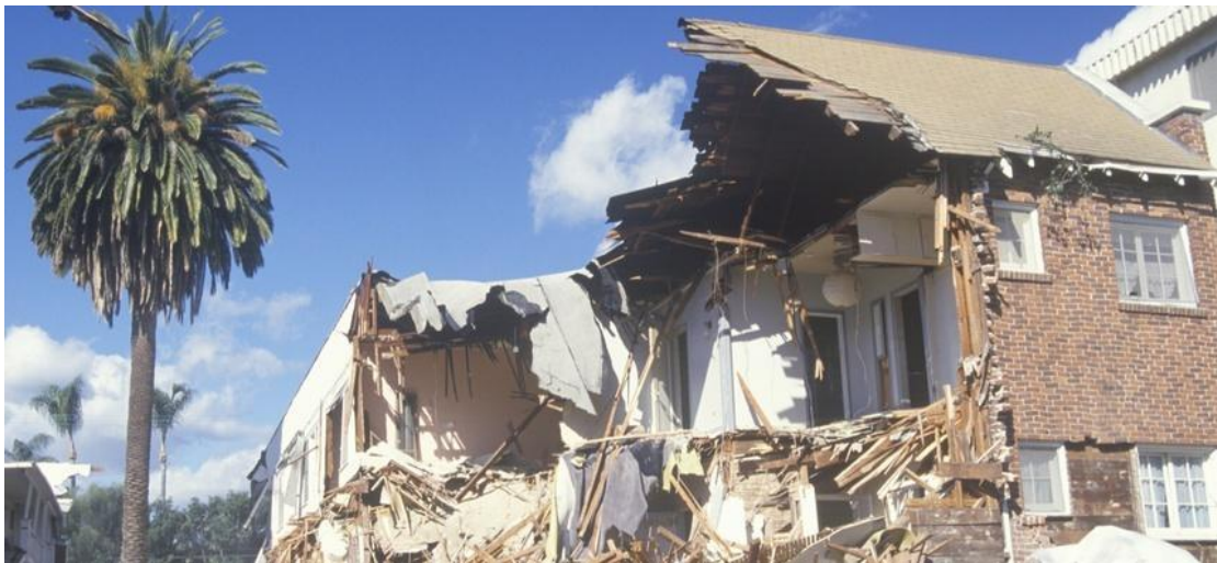
Damage from the 1994 Northridge earthquake in Santa Monica, California
